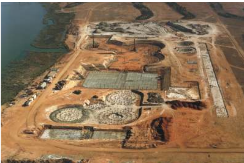
New Treatment Station Foundations (Huelva)
