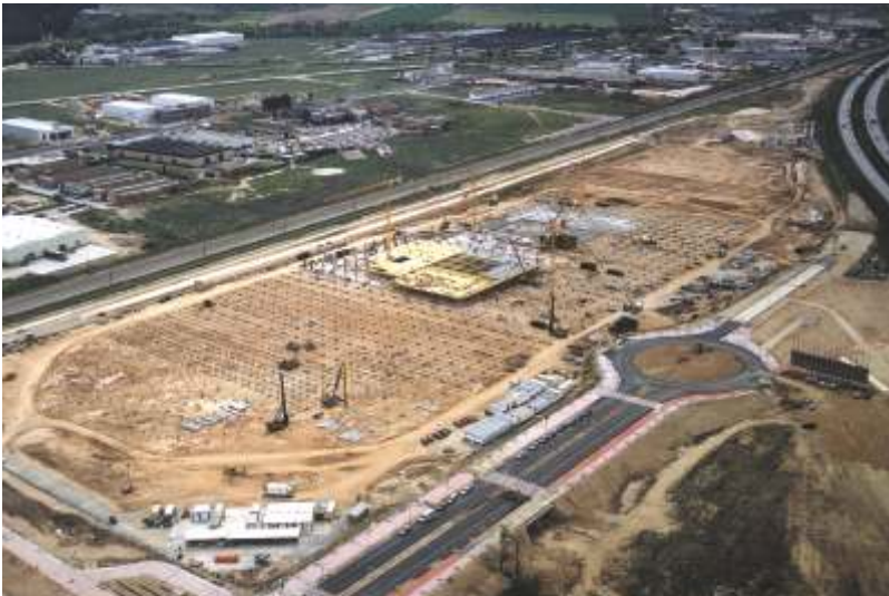
"HIPERCOR" Shopping Centre Foundations, La Garena (Madrid)
