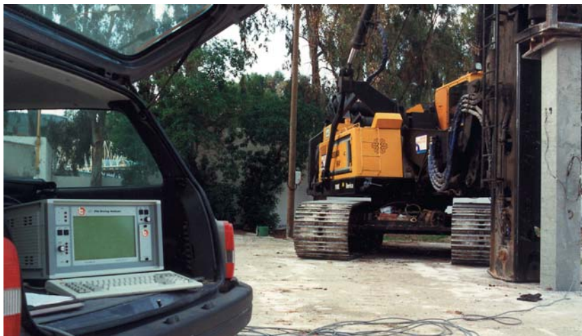
Trial with the pile drive analyser
