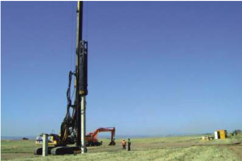
Foundation for a Thermosolar Plant in Palma del Rio (Sevilla)
