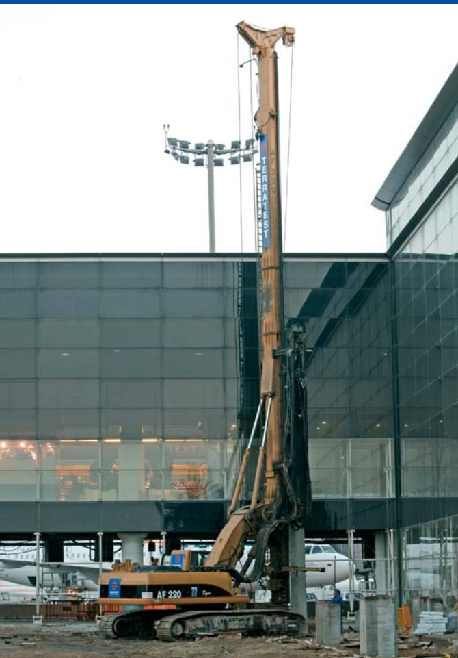
Terminal A Extension Barcelona Airport
