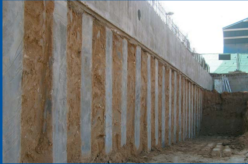
Pre-tensioned Pre-cast Piles Curtain, Alcobendas (Madrid)
