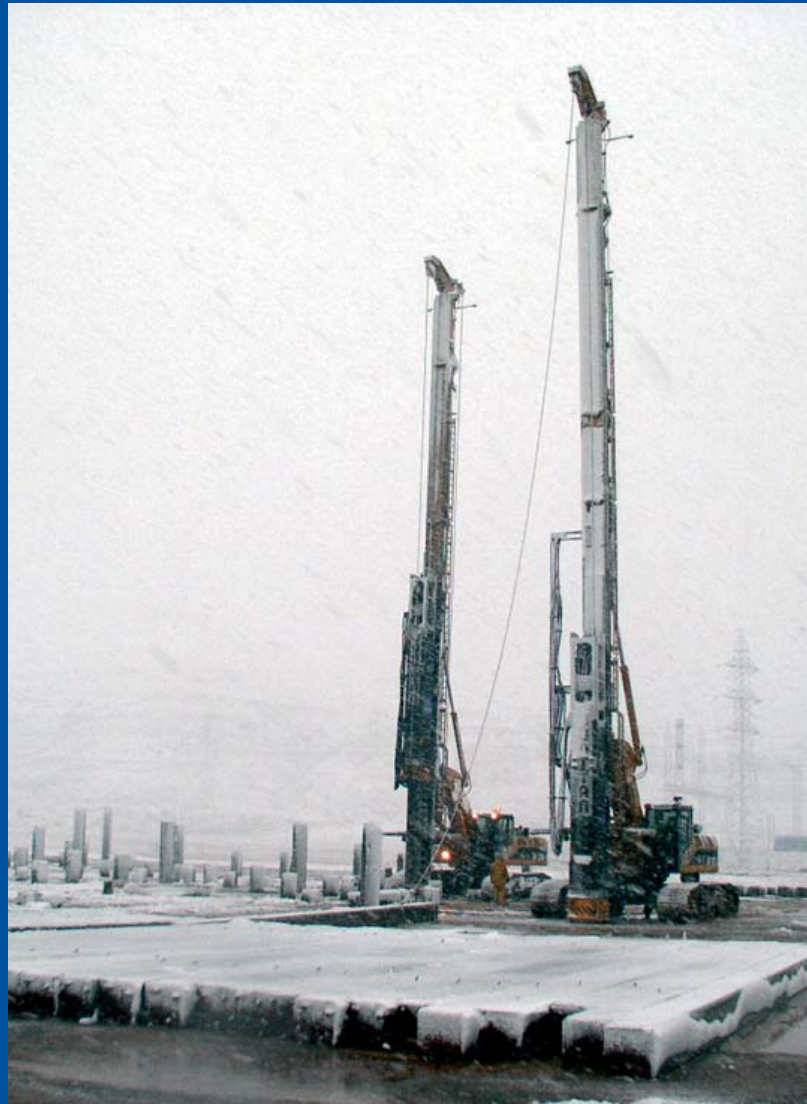
Arrubal Combined Cycle Power Station Foundations (La Rioja)
