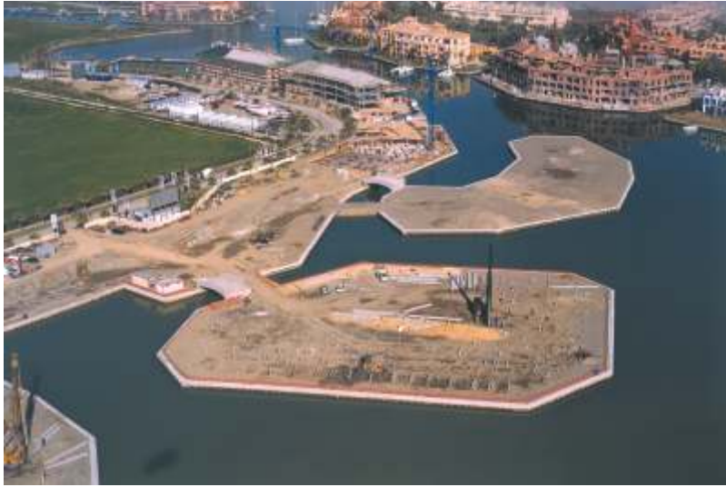
Foundations for apartment building, Sotogrande (Cádiz)
