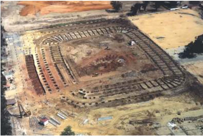
New Colombino Stadium Foundations (Huelva)
