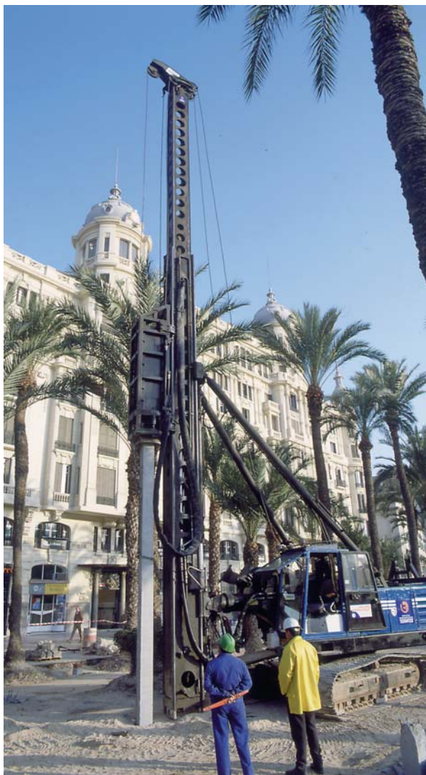
Foundations for the España Esplabade in Alicante
