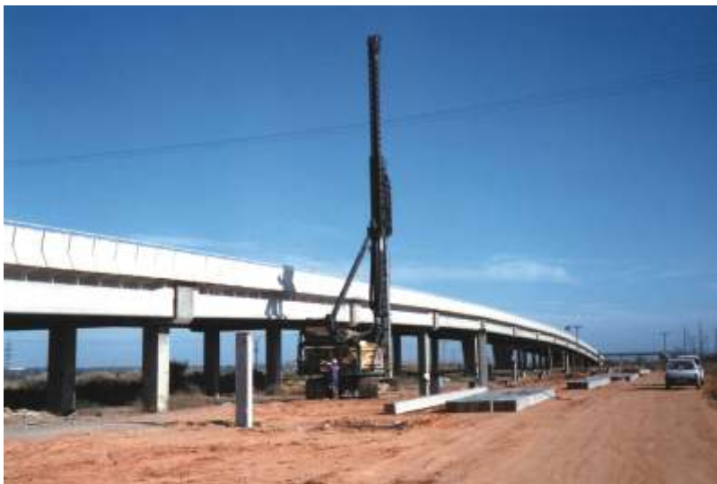
Enlargement of structures on the Southern Ring Road (Huelva)
