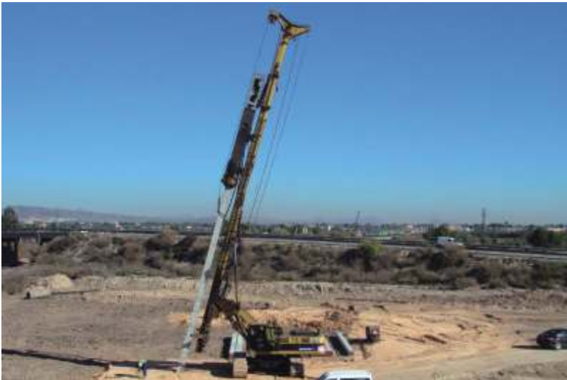
Foundation by Precast Pile on Crevillente Hig Speed Railway at (Alicante)
