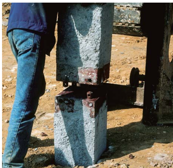
Phase 1: Placing the pile for joining
