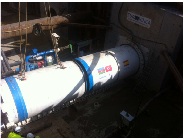
Airlock connection works during first drive.
