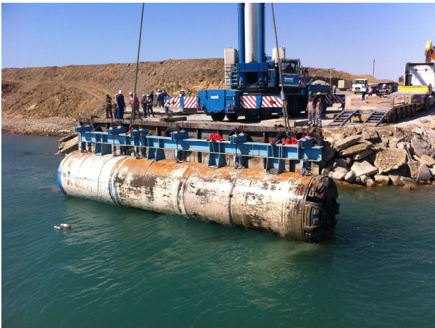
Rescue final stage, TBM is taken on-shore.
