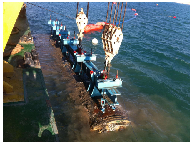
TBM lifted by barge's crane during rescue stage.
